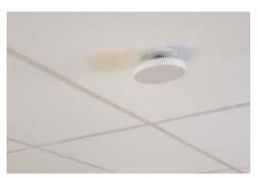
The Dual Band Dot, part of the Ericsson Radio Dot System, enables a simple deployment that is fully integrated with the outdoor macro network. The Dual Band Dot enables multi-band deployments and Carrier Aggregation, which is important in 5G readiness.
