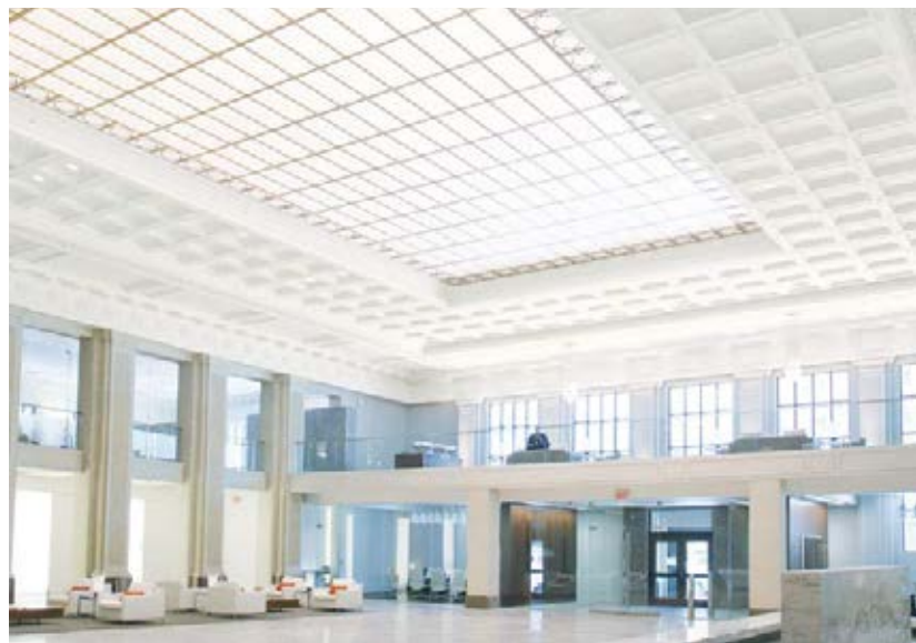
▲ Plasterform™ GRG coffers and cornice; The Rockwell Building, Cleveland, OH Sandvick Architects and Vocon
