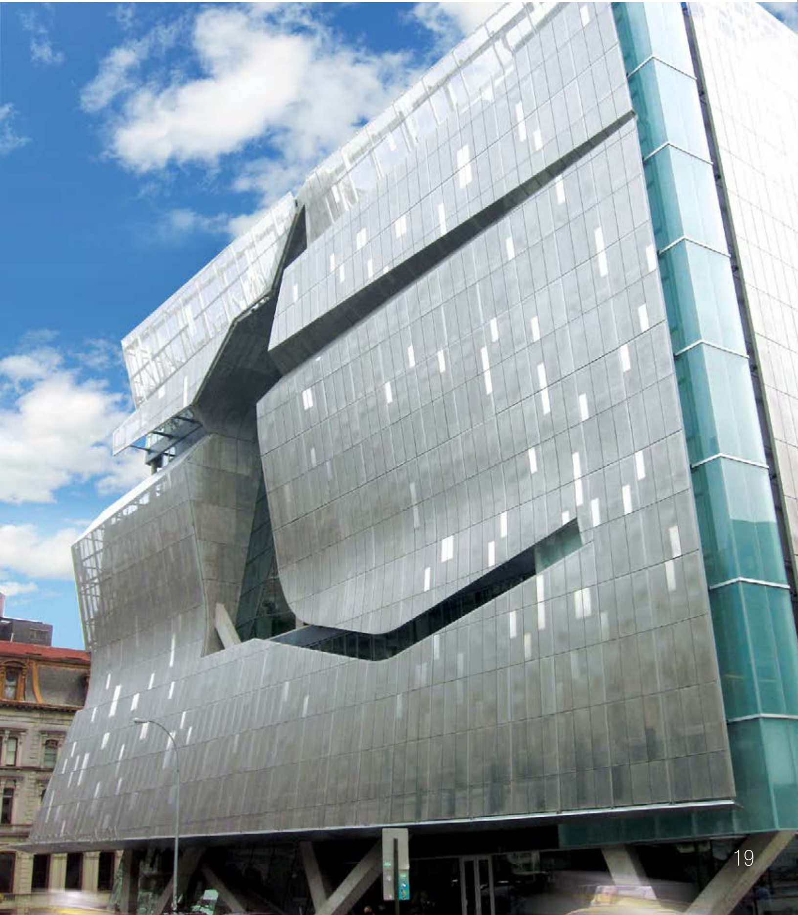
▼ Plasterform™ GFRC rainscreen panels; The Cooper Union, New York, NY; Morphosis
