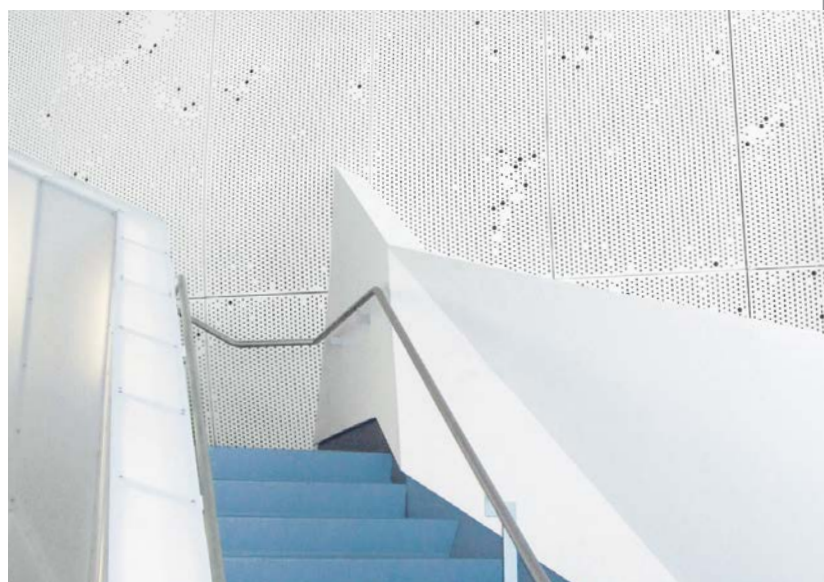
▲ Plasterform™ GRG randomly perforated sound absorbing panels The Cooper Union, New York, NY; Morphosis
